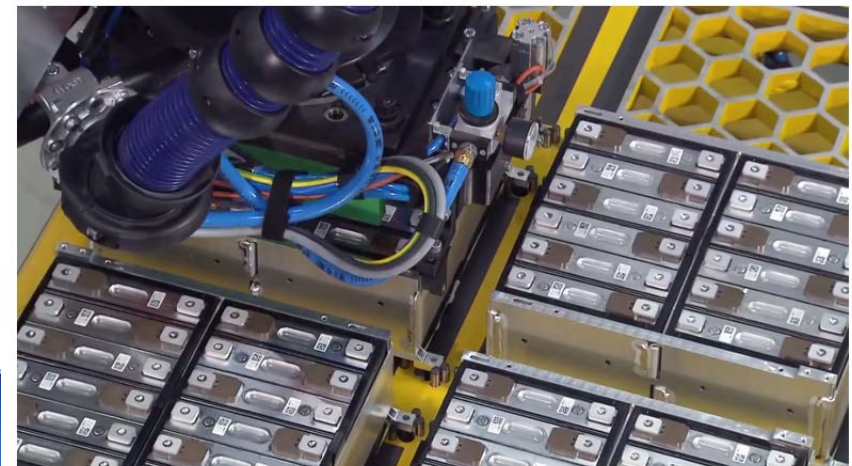
FIGURE 1.26 BMW I3 BATTERY MODULE
